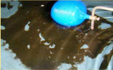
Moderate fouling suggesting cleaning should be conducted during the next 12 months
