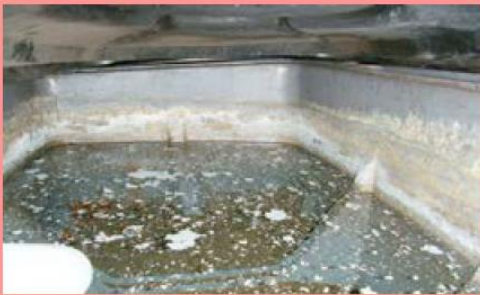
Unusually heavy scale formation requiring more than a regular clean and disinfection
